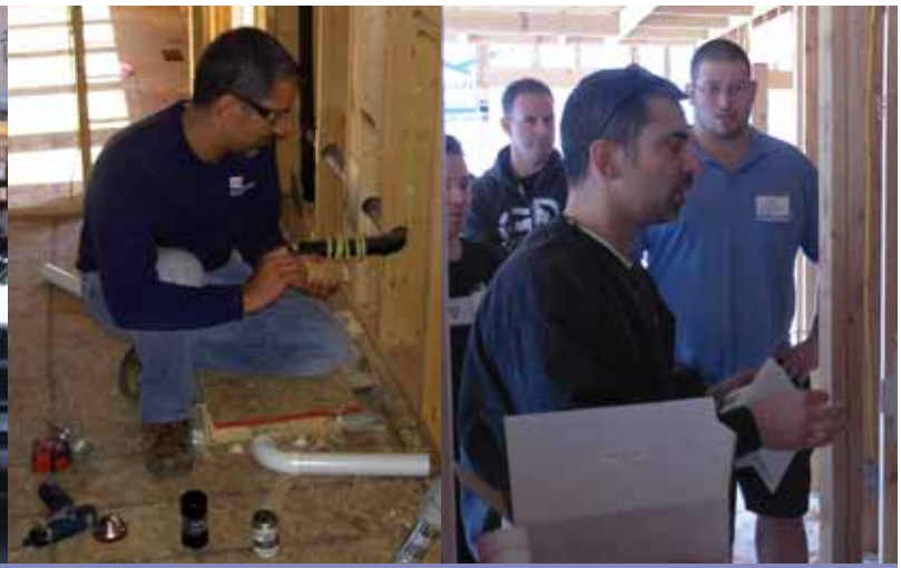
(above) The 2010 Installation Seminar participants outside the new construction site. (center) Chris Slackford, Training Manager for H-P Products, performs the rough-in for the Vroom quick-clean hose management accessory. (right) Chris Slackford, Training Manager for H-P Products, explains the installation process for Hide-A-Hose Hose Management System.
