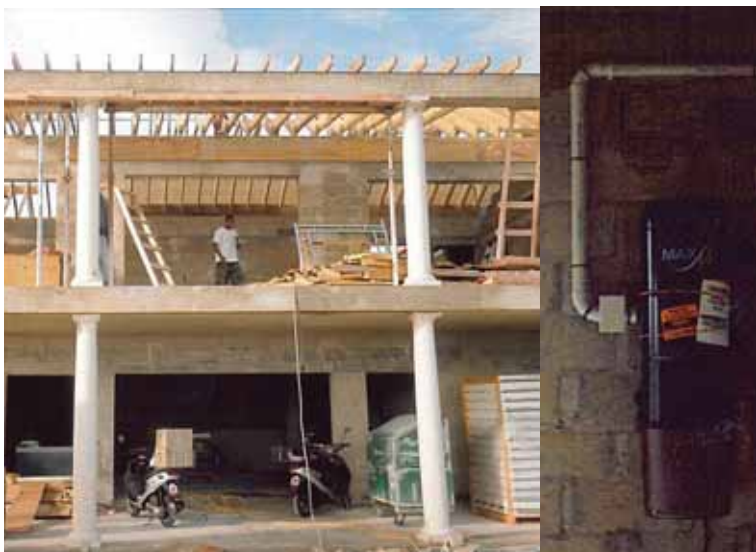
(above) The home was a 13,000 square foot, two-story, cement structure. (right) The VACUFLO® MaxAir power unit was installed to run the whole system.
